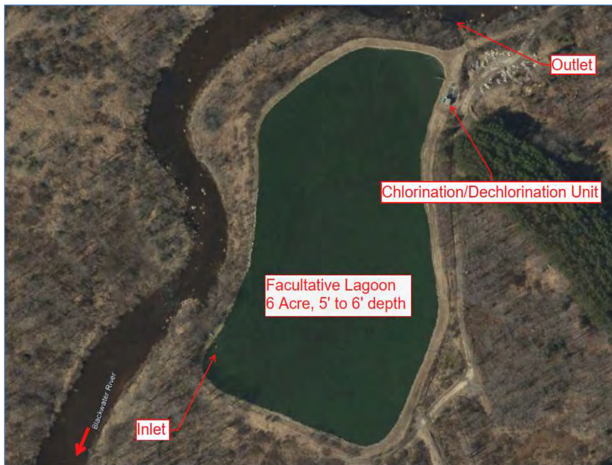
Figure 2 - Town of Davis WWTP
